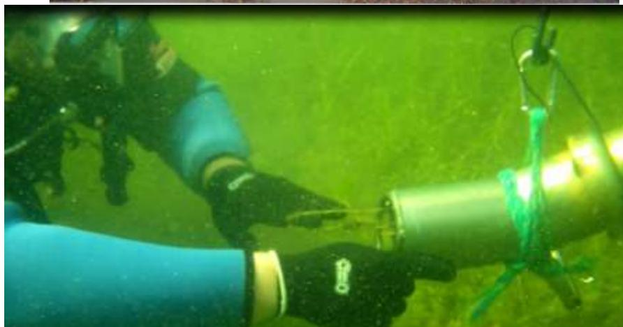
Figure 68: DASH - Diver Assisted Suction Harvest (Aquacleaner Environmental, <http://www.aquacleaner.com/index.html>); Many Waters, LLC)
